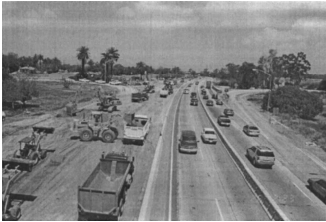
Fig. 2. Around-the-clock construction operations and counterflow traffic with MCB
